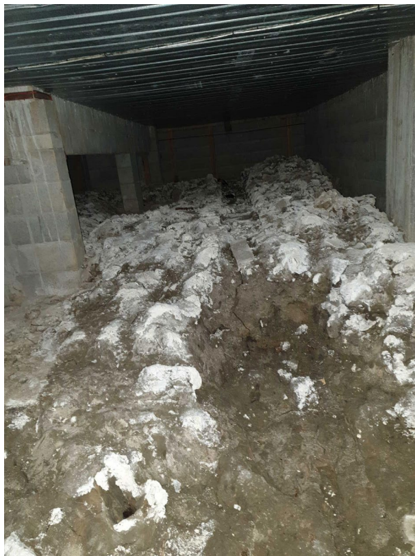
Figure 33 - Efflorescence is present indicating dampness from a subterranean source is evaporating into the subfloor space
