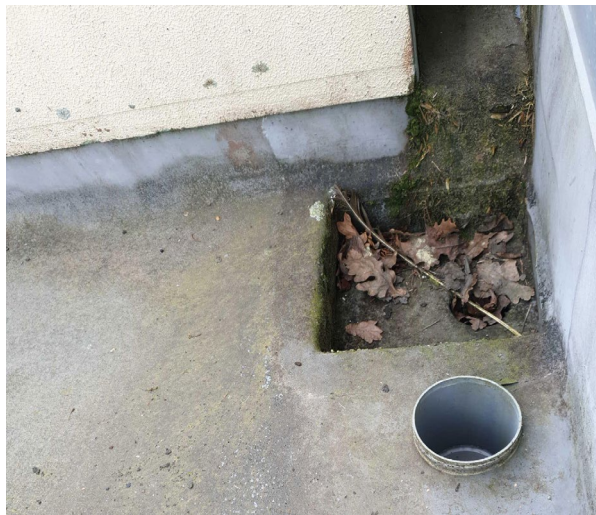
Figure 52 - organic debris in the rain head
