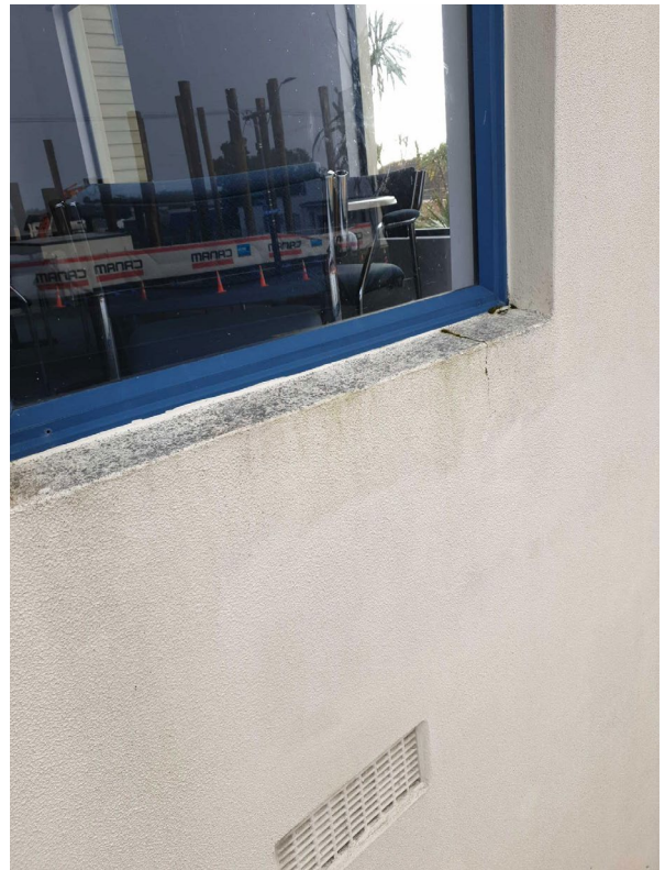
Figure 55 - no sill flashing
