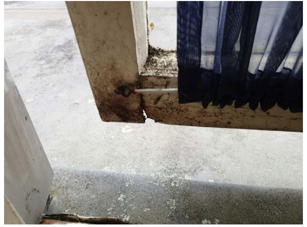
Figure 10 - The joinery has significance fungal deterioration and mould growth
