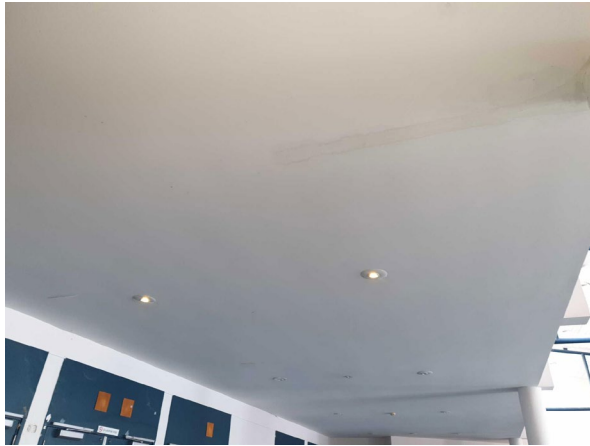
Figure 17 - Water damage to some of the ceiling plasterboard
