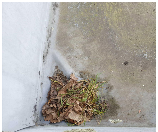
Figure 51- organic debris is blocking some drains
