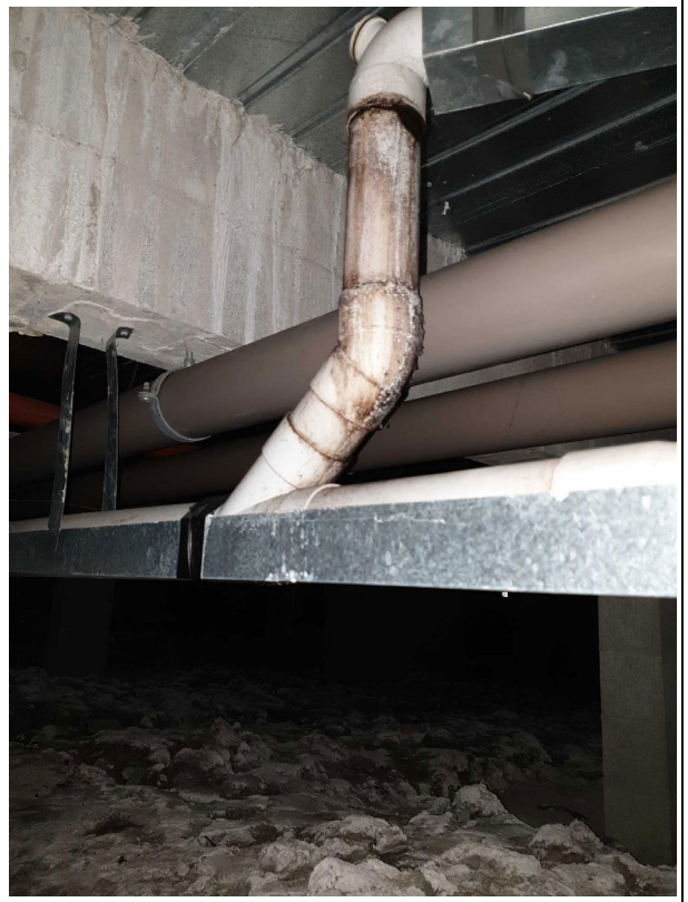
Figure 34 - The sewerage riser is leaking and should be attended to urgently
