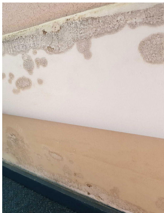
Figure 4 - Water damage and mould to the backside of vinyl paper and plasterboard
