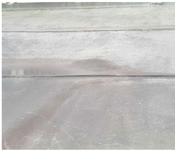
Figure 50 - the laps of the waterproofing membrane are counter to the rake and water is able to push into the joint.
