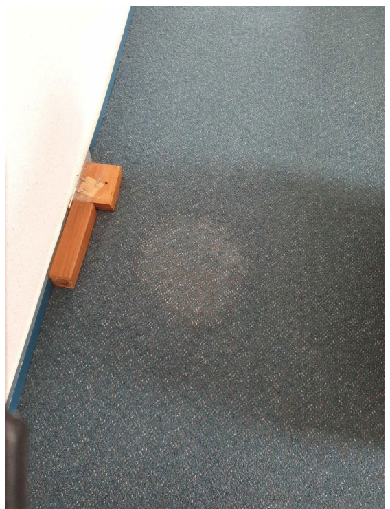
Figure 8 - Spots of visible mould on the carpet
