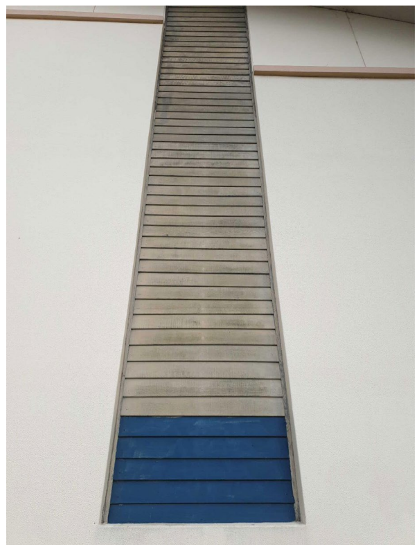
Figure 57 - the weatherboards require treatment with wood preservative
