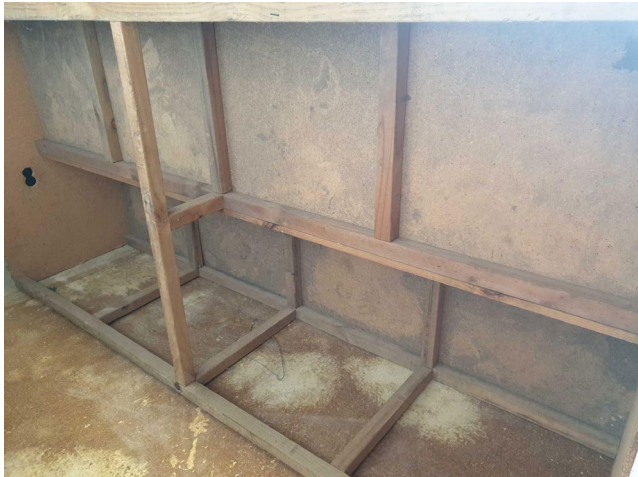
Figure 43 - Some staging that is kept in the storage is unsalvageable and will require disposal
