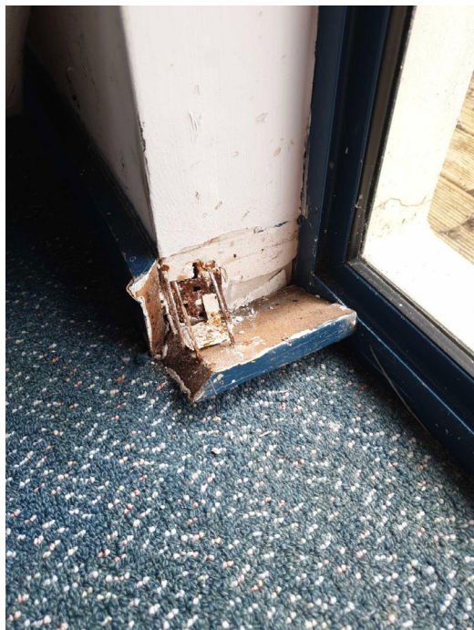
Figure 1 - Mould and elevated moisture levels on skirting boards, lower wall linings and carpet
