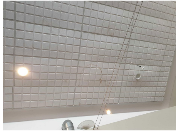
Figure 18 - Water damage to some of the ceiling tiles
