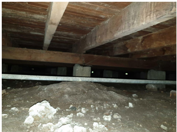
Figure 35 - The bottom side of the floor boards and some isolated areas showing signs of visible mould growth
