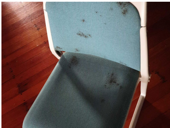
Figure 11 - Some of the soft furnishings were found to be significantly damaged by mould
