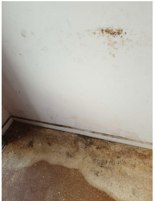
Figure 42 - The growth has affected skirting boards, lower wall boards and the floor in some areas
