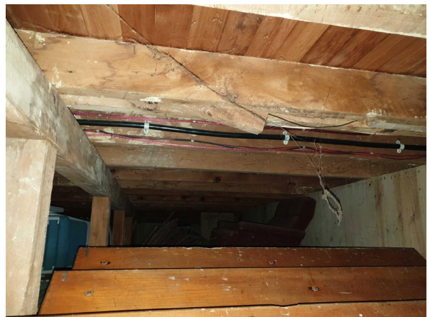
Figure 12 - The underside of the stage showed signs of water staining and topical fungal growth
