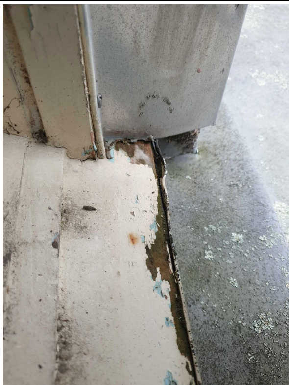
Figure 45 - there are no sill flashings along the top of the gymnasium
