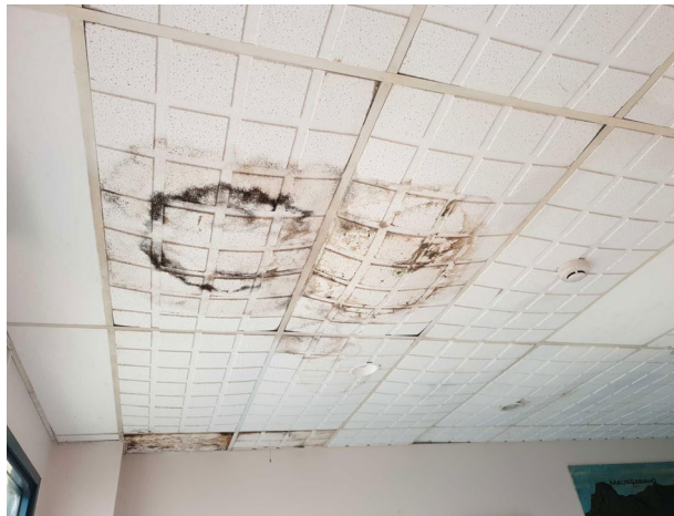
Figure 27 - Heavy growth on some of the ceiling tiles
