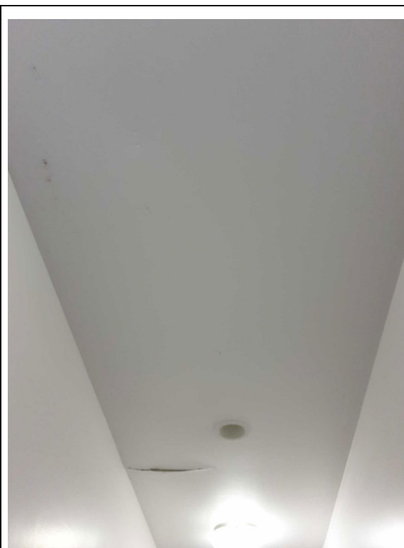
Figure 23 - Water damage to ceiling
