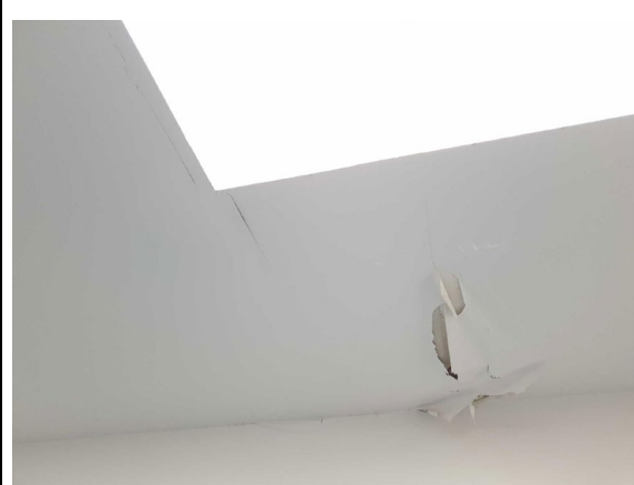
Figure 25 - Water damage to ceiling
