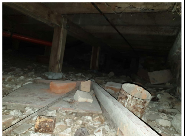
Figure 36 - Building rubble and debris is growing visible mould from the damp surroundings
