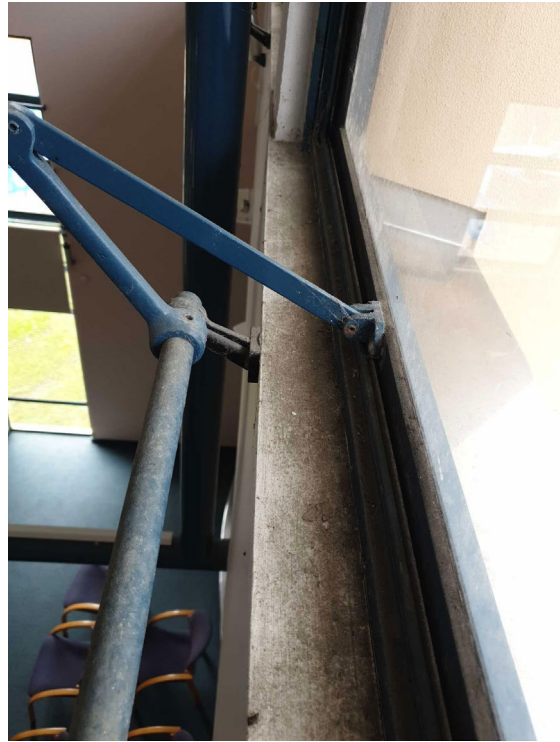
Figure 5 - Superficial mould to the window sills
