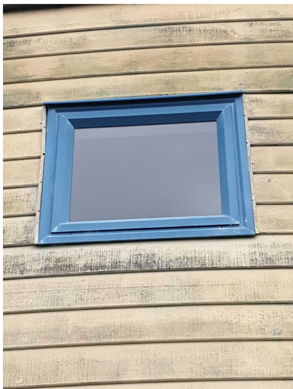
Figure 56 - the weatherboards require treatment with wood preservative
