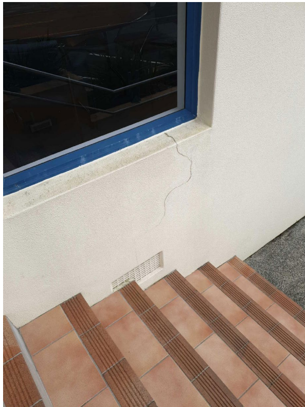
Figure 54 - step cracking in the render
