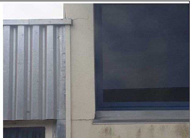
Figure 59 - cracking in the render
