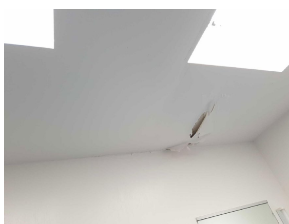
Figure 26 - Water damage to ceiling and wall
