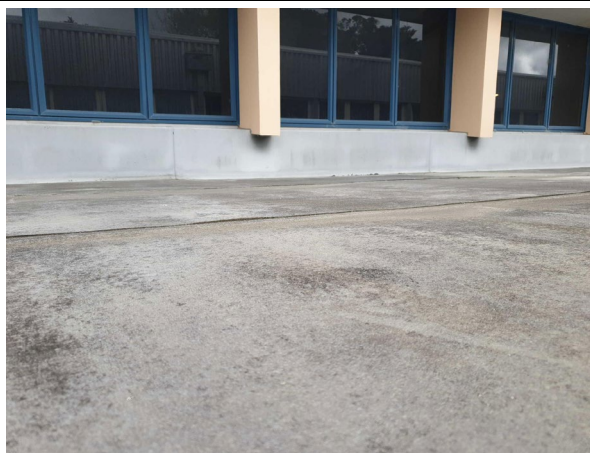
Figure 47 - there is inadequate fall
