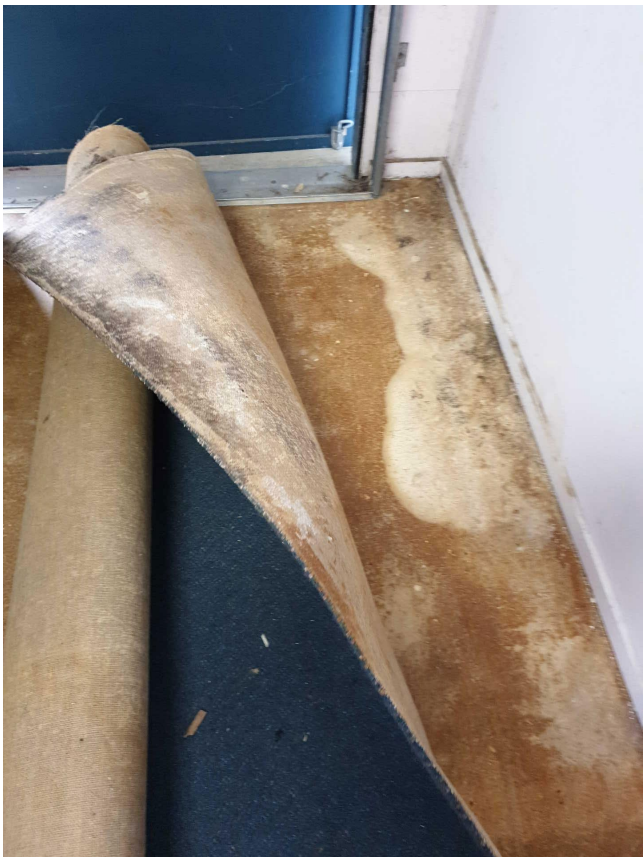
Figure 41 - Visible water damage and mould growth to the top and bottom of some of the carpet storage
