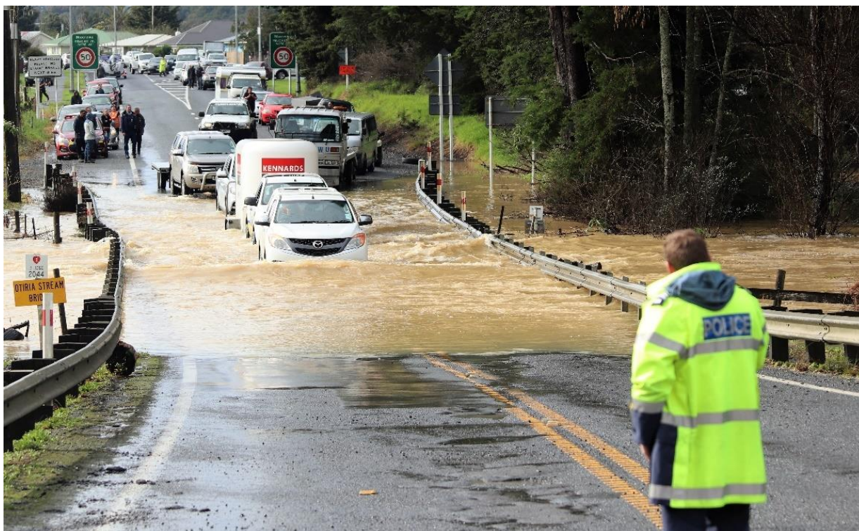
Turntable Hill flooding
