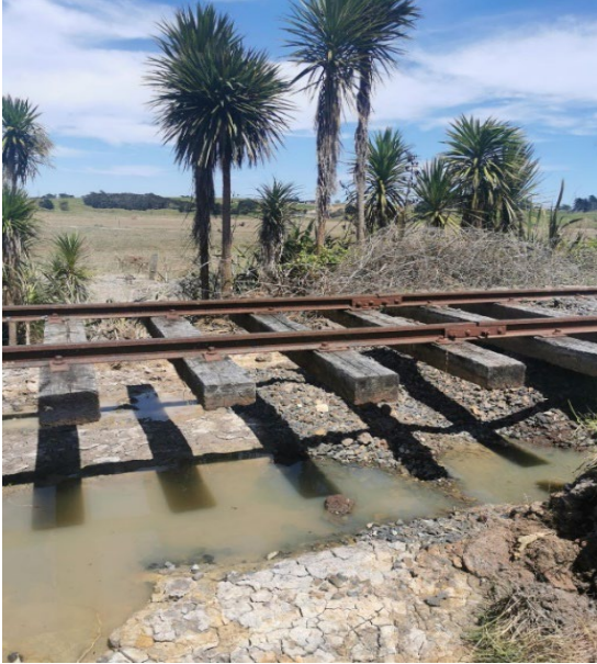
Figure 10 - Awakino Valley Railway embankment eroded, overtopping, and affecting the Dargaville wastewater treatment plant
