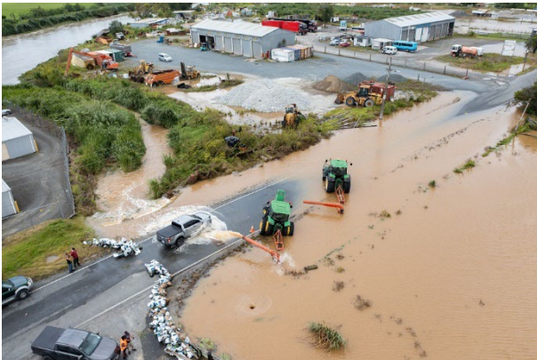
Figure 16 - Flood pumps on Beach Road pumping flood waters to the Kaihu river
