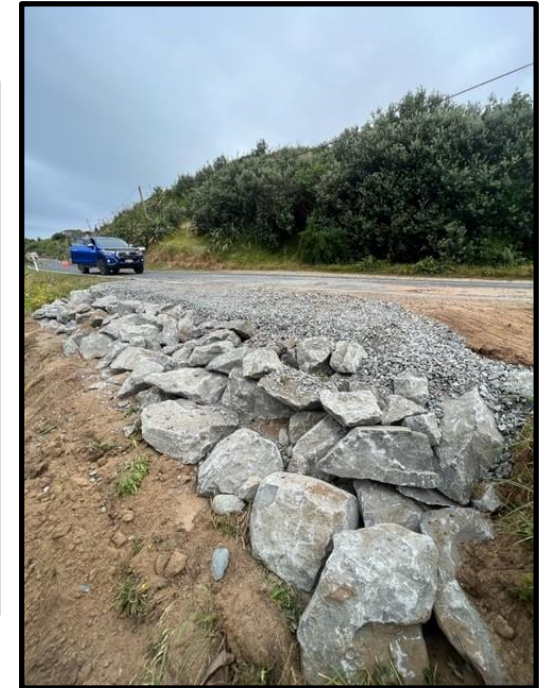
Glinks Rd, shoulder repair.
