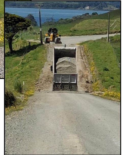
Some of the unsealed road works carried out in Dec 2024.
