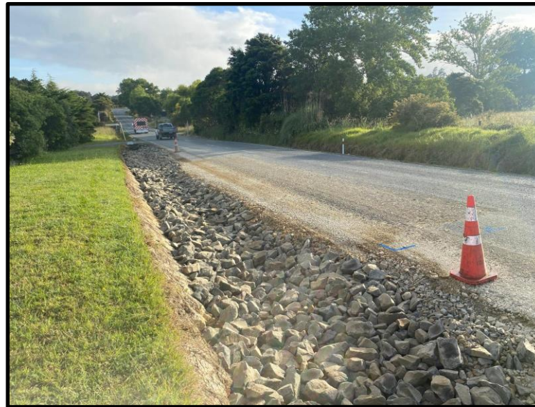
Sealed Maintenance on Kaiwaka-Mangawhai Rd. Digout & water table/shoulder reconstruction.
