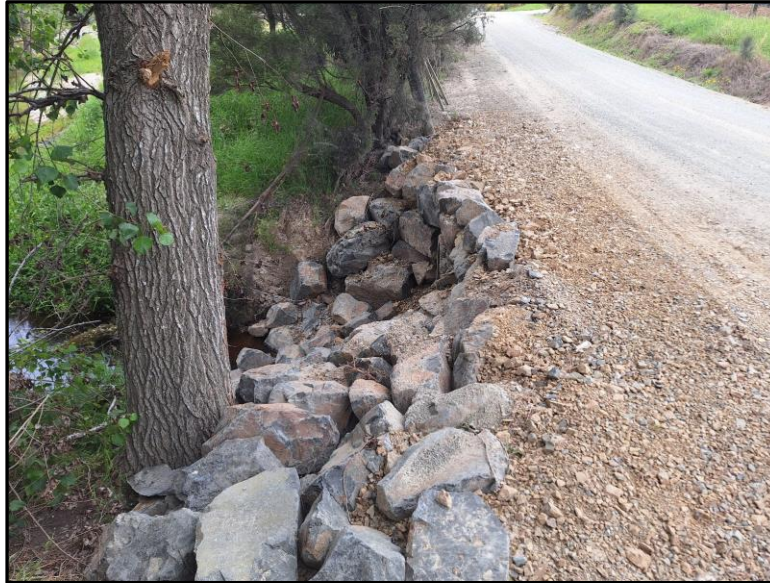
Above-Works on Kapawiti Rd.
