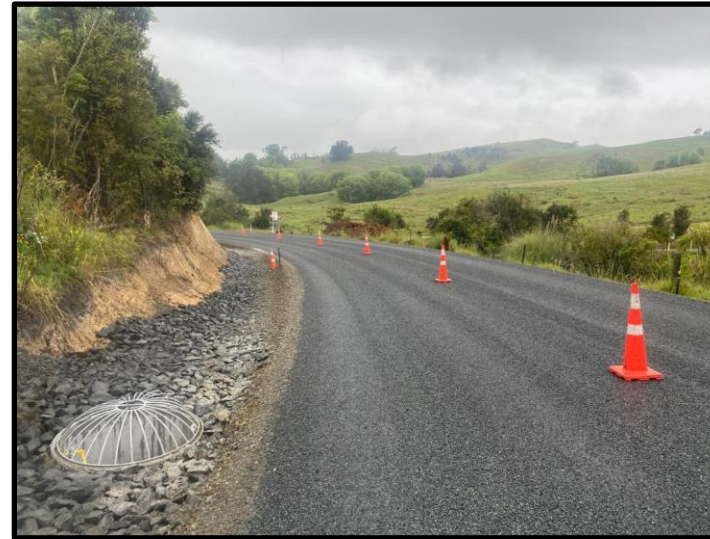
Chip seal on Whakapirau Rd Rehab site.
