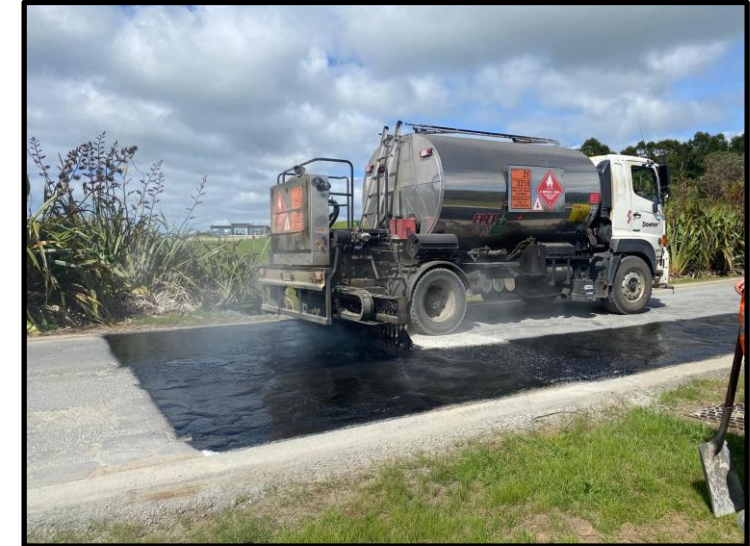
Pre-reseal repairs Cames Rd.
