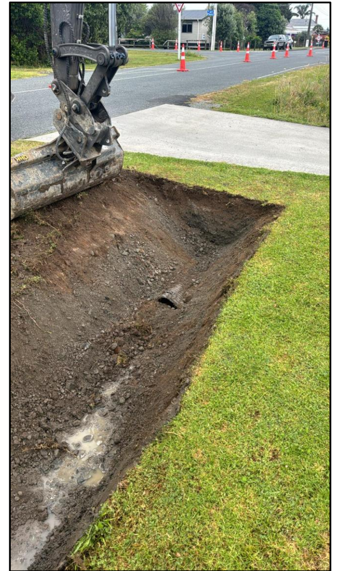
Above – water tabling works during Dec 2024
