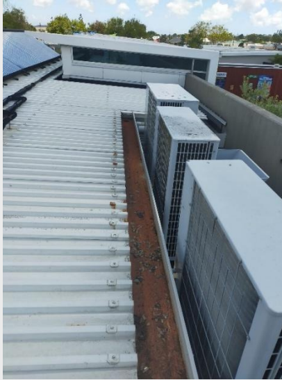
2.2. Roof gutter rusting
