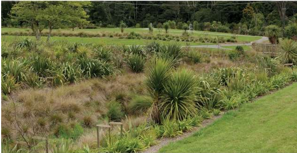
Figure 3: This image shows a swale planted with native plants.
