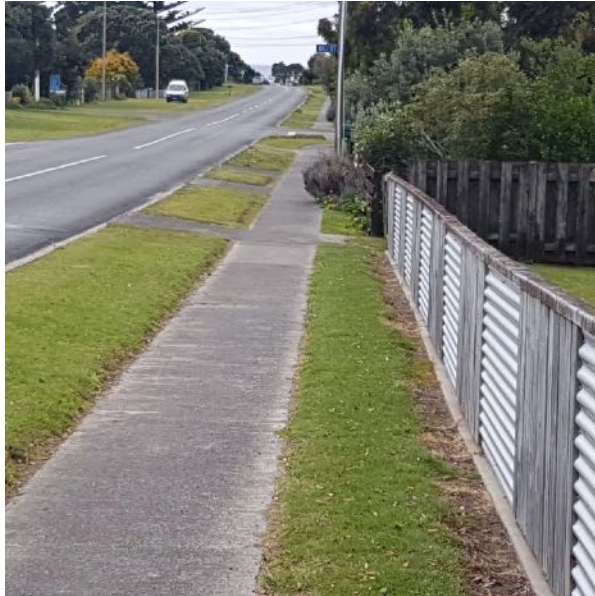
North Avenue, existing height of foot path precludes widening towards kerb
