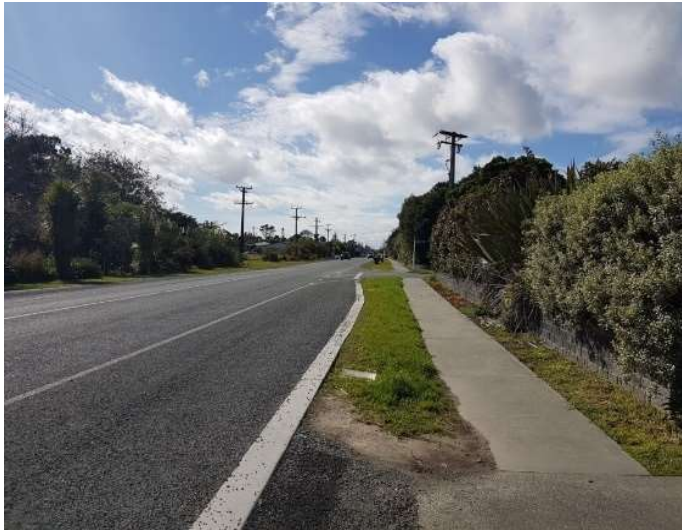
Moir Street; Existing RHS footpath is below kerb level
