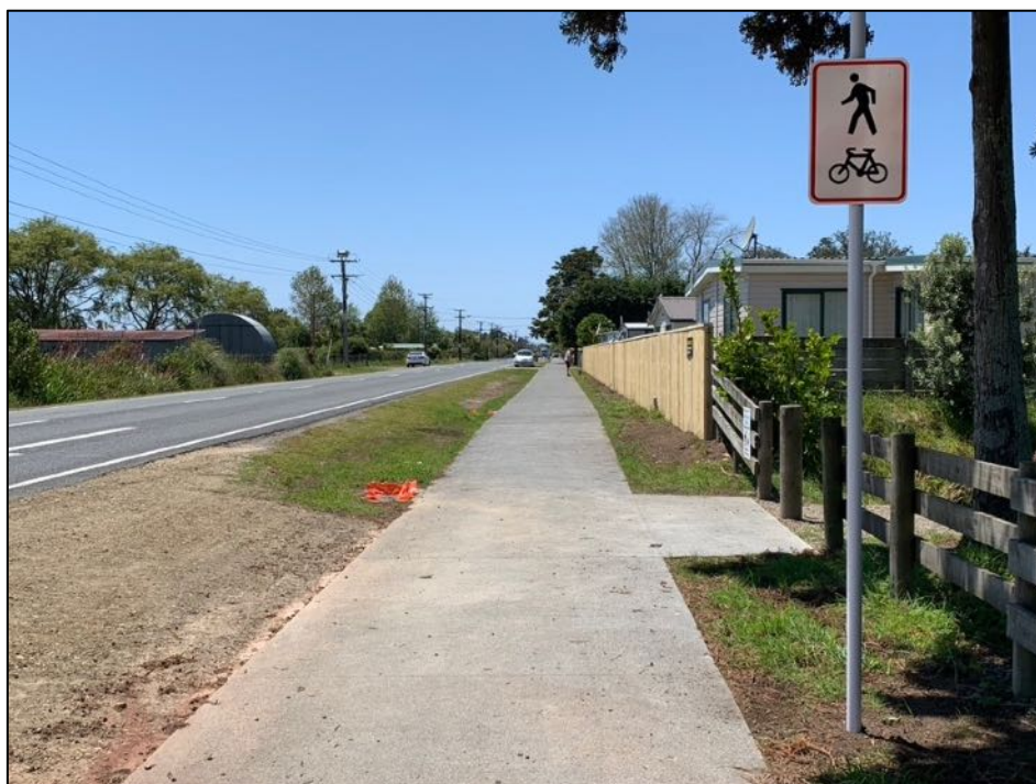
Figure 2: The new 2.5m local shared path connection along Moir Street in Mangawhai Village that was constructed in early 2019.
