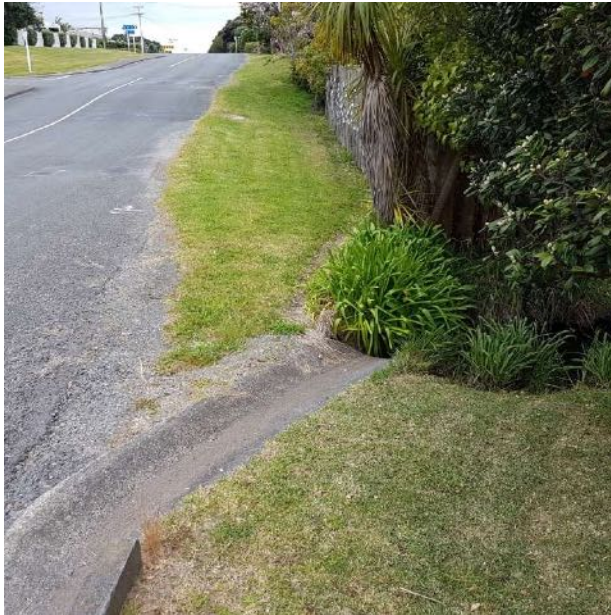
RP 250, 900mm culvert to be extended
