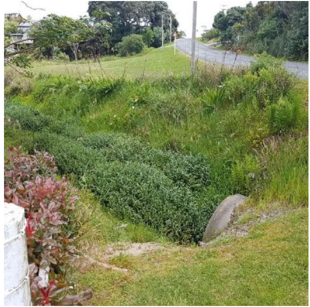
RP 490, 1200mm culvert to be extended
