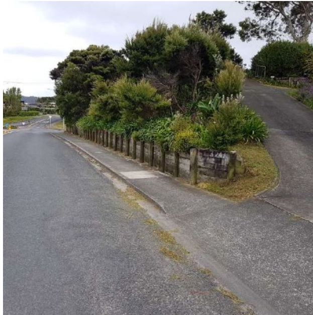
Molesworth Drive: the existing retaining wall RP 4955 to 4995 to be replaced with 2.5m height wall to provide for the proposed 2.5m shared path
