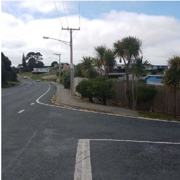
Mangawhai Heads Road West: South side constraints to widening existing foot path
