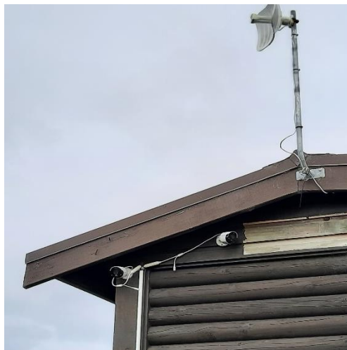
Arlo CCTV system (2 cameras only)
