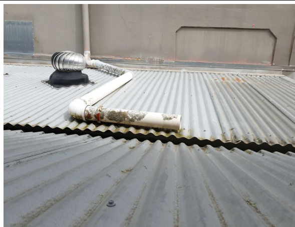
Figure 48 - the discharge from the upper roof does not disperse well
