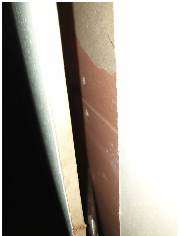
Figure 16 - Double lining appears to be standard with Plywood then Fireline being the 2nd layer
