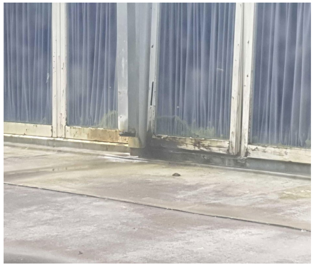
Figure 53 - some window joinery has signs of serious deterioration and cannot close.
