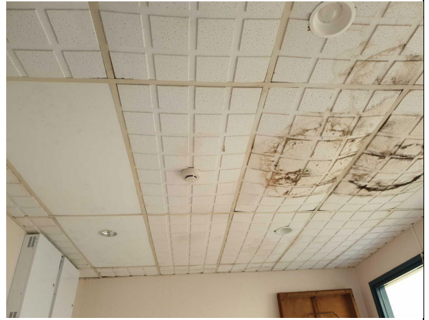
Figure 28 - Heavy growth on some of the ceiling tiles
