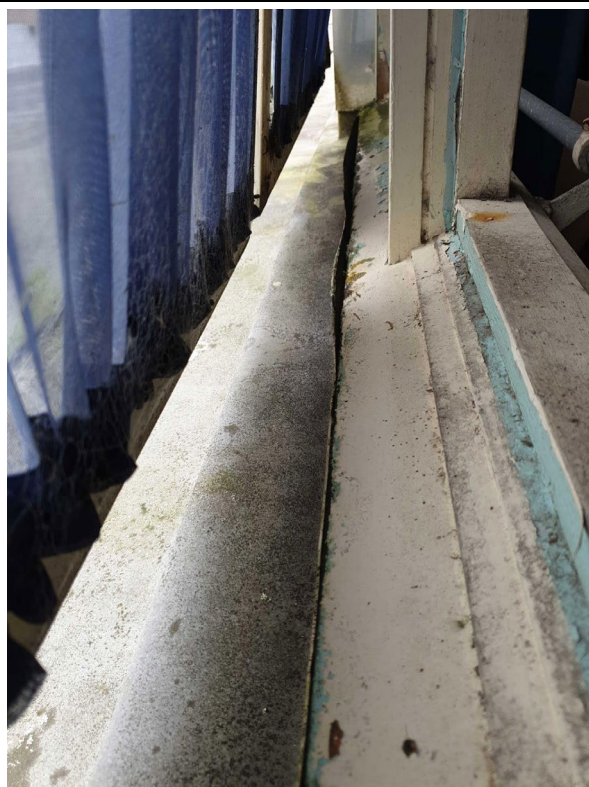
Figure 46 - the water proofing membrane does not turn up behind a wet or dry flashing
