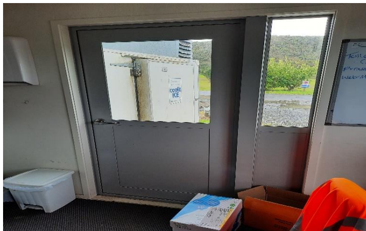
Rear office door
