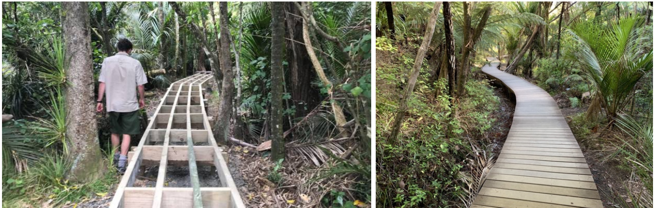
Figure 3 - Photographs showing construction of and finished boardwalk at Kitekite Falls, Piha - design specifically for PA.
