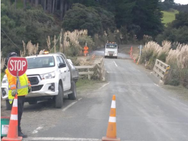
Pouto Road Sealing
