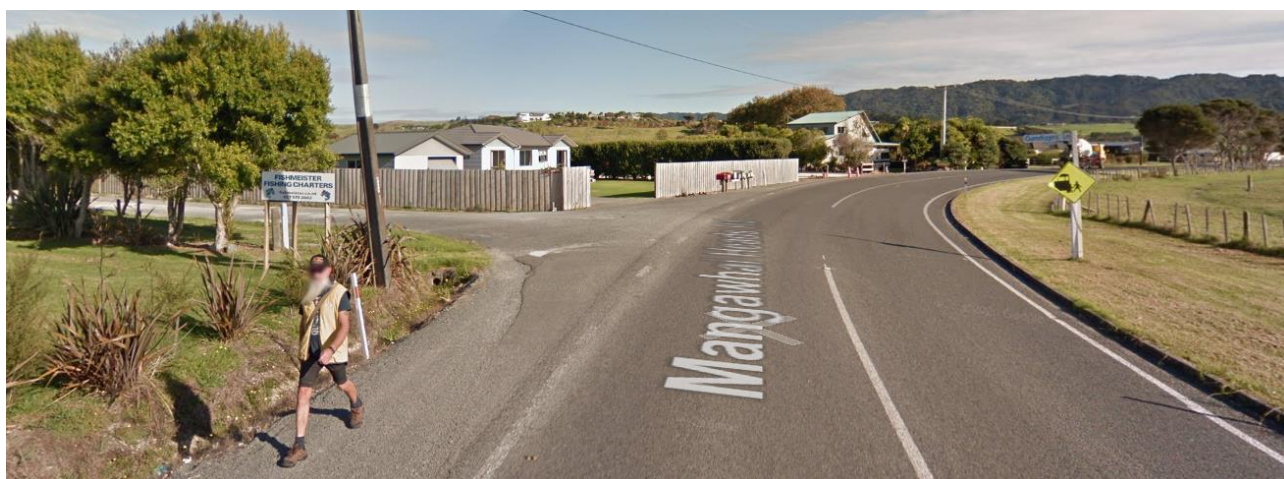
Figure 27: Mangawhai Heads Road (West) – 70kph zone showing lack of pedestrian facilities and direct access residential dwellings.
