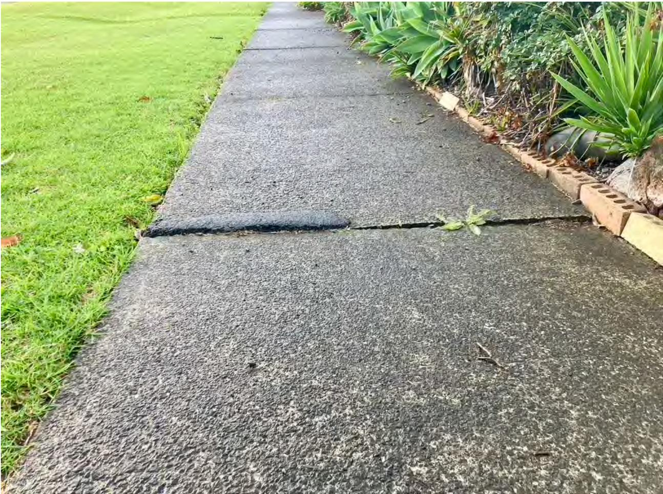
Tar snakes in Liverpool Street Dargaville where there are un-remediated cracks in the road adjacent to filled cracks. This is the situation in quite a bit of Liverpool Street between Logan Street and Colville Road.
