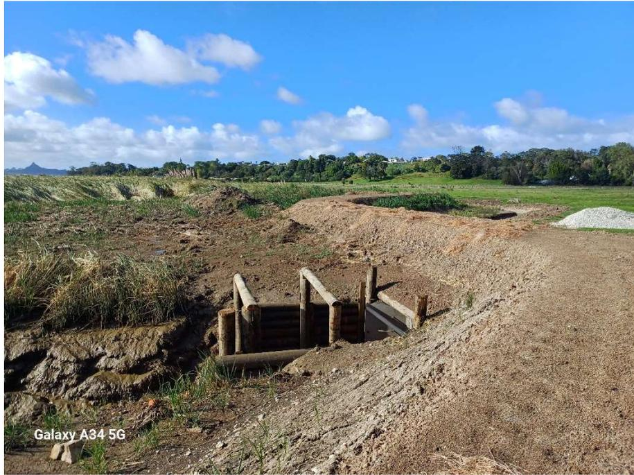
Replacement floodgate unit installed in Rope's property in February
